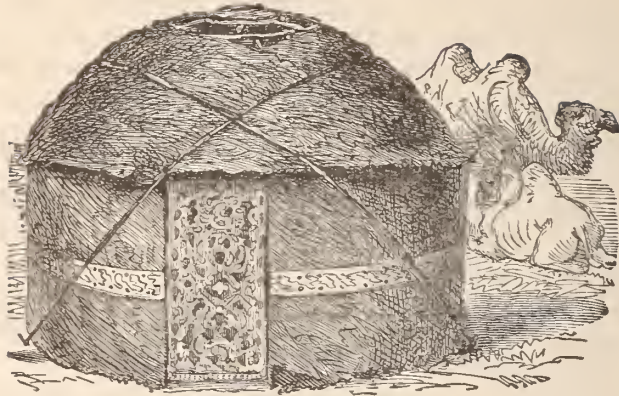
TENT, AS COMPLETED.
